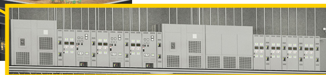
Transfer Switches and Power Control Switchgear
